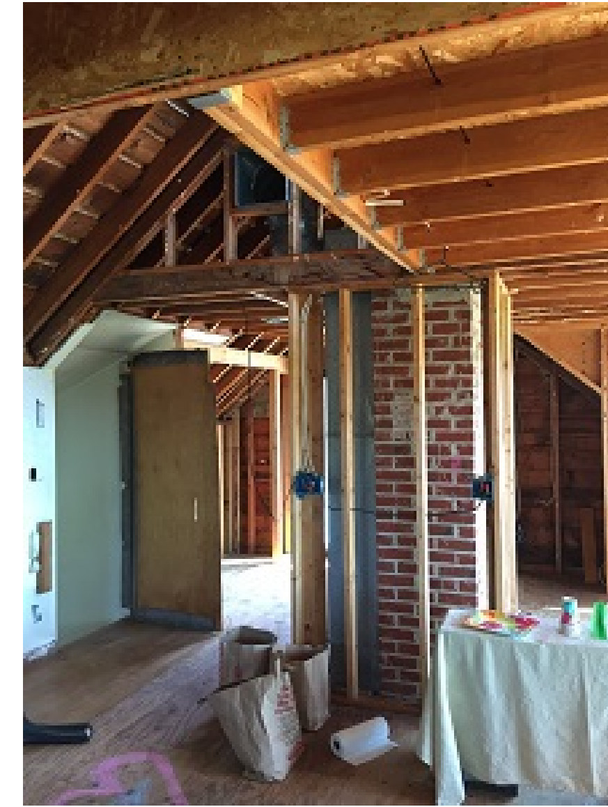
NOTE CHIMNEY AND CEILING FRAMING
