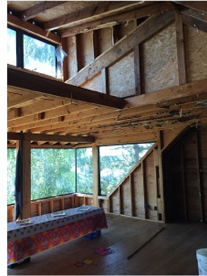
NOTE DORMER AND ROOF FRAMING
