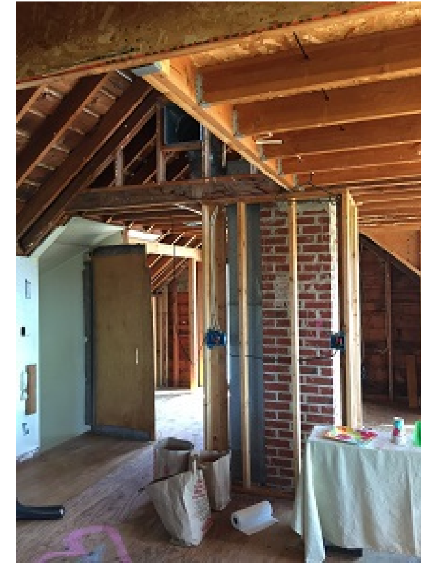
NOTE CHIMNEY AND CEILING FRAMING
