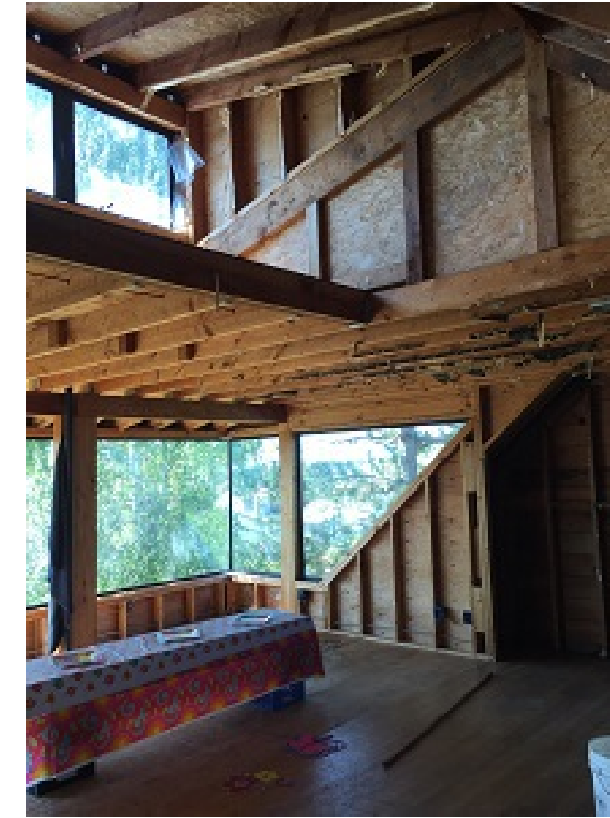
NOTE DORMER AND ROOF FRAMING
